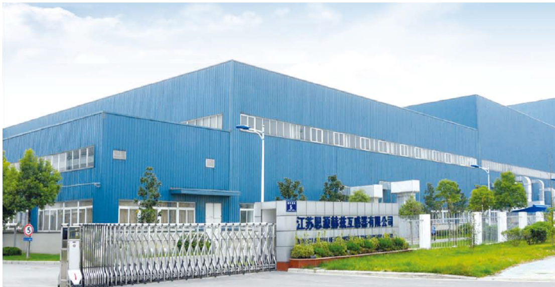
Figure 1-1 Sieyuan Hertz Instrument Transformer Co., Ltd
