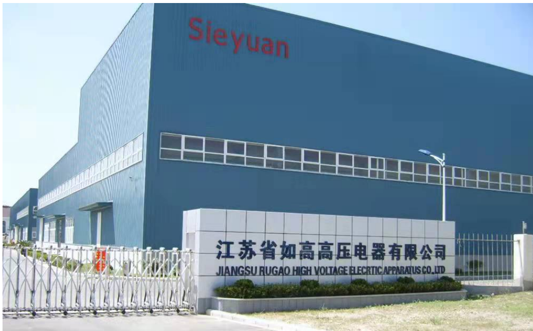
Figure 1 Jiangsu Rugao High Voltage Electric Apparatus Co., Ltd
