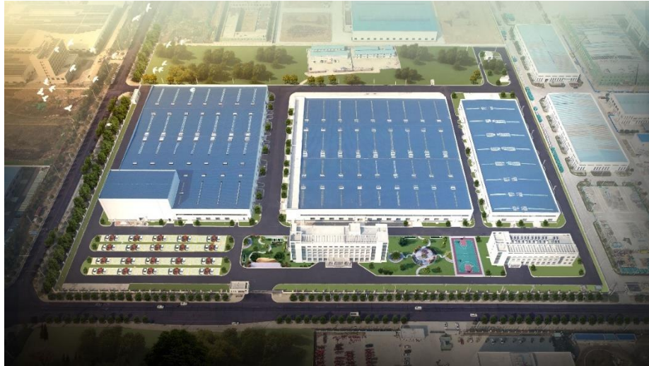
Figure 1.1.1: Aerial view of Xiangyang Guowang
